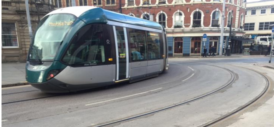
Figure 3-2: Nottingham Express Transit (NET) - Tram Track
