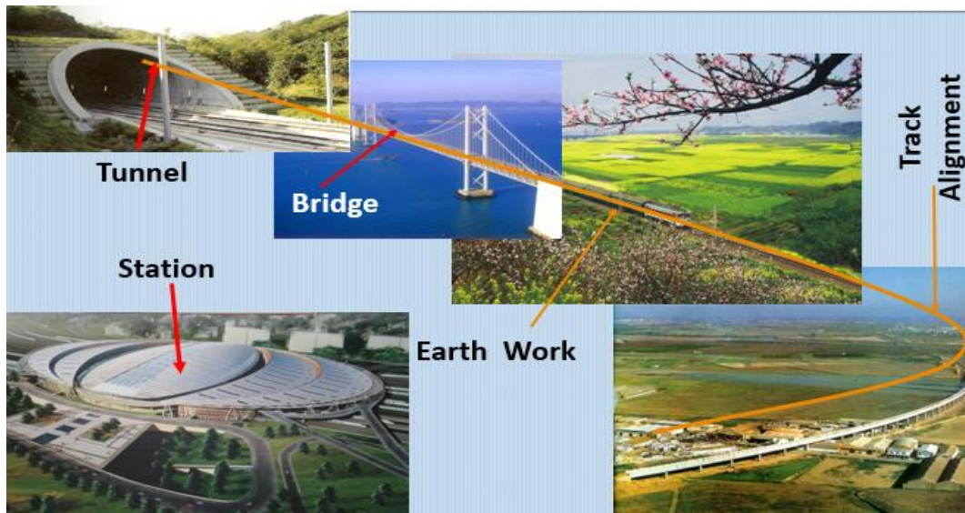
Figure 1-7: permanent infrastructure of railway
