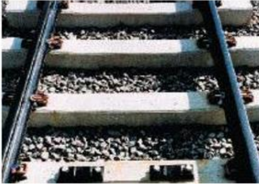
a) Mono-block concrete sleeper
