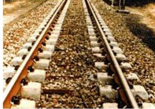
b) Twin- block concrete sleeper
