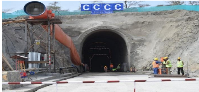
Figure 4-1: The tunnel works at Weldiya-Mekelle railway project
