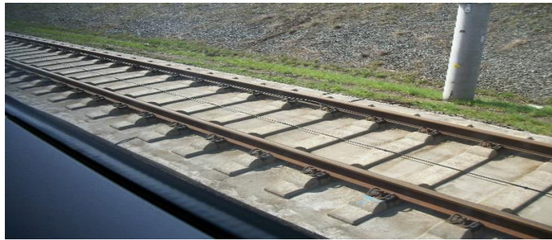
Figure 3-3: Fiber Reinforced Concrete Slab Track
