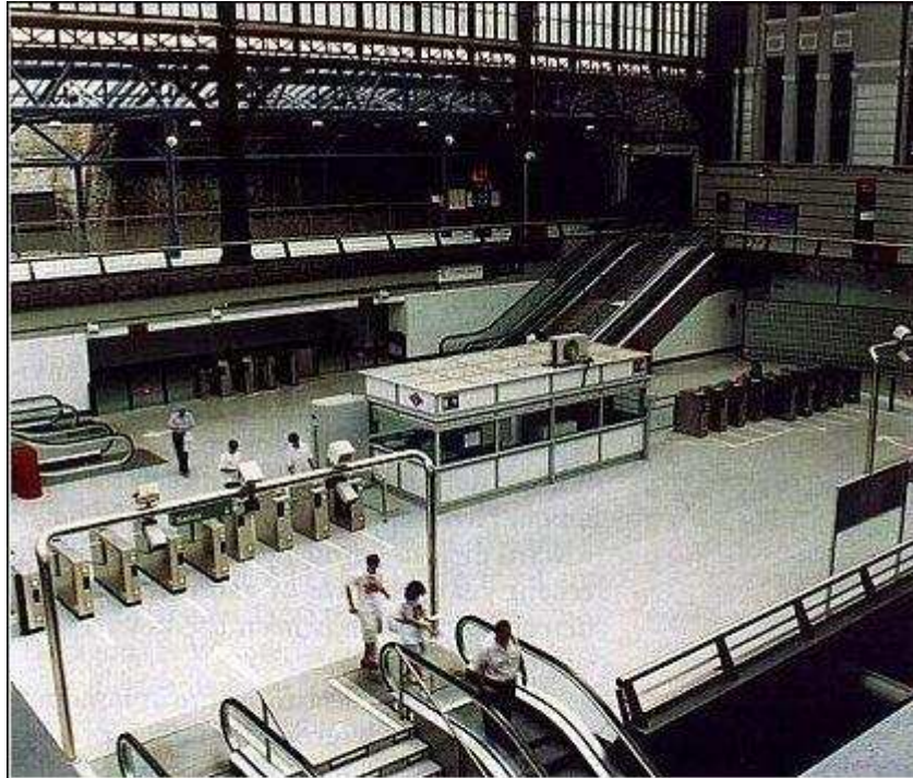
Madrid, Spain, offers an example of a light, airy station concourse with faregate lines dividing the "paid" and "unpaid" areas. The ticket office is located in the centre of the gate line so it can be used by passengers in both areas. The lightweight steel structure over the escalators in the foreground carries CCTV cameras and loudspeakers.
