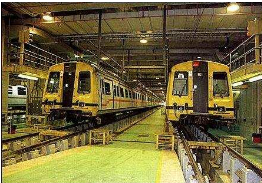
Interior of inspection shed at Ho Tung Lau, KCRC Hong Kong, showing "swimming pool" layout of floor with trains standing on rails mounted on concrete posts to give underfloor access. Note also the roof level walkways on the outside of the trains to give access to pantographs and air conditioning units.
