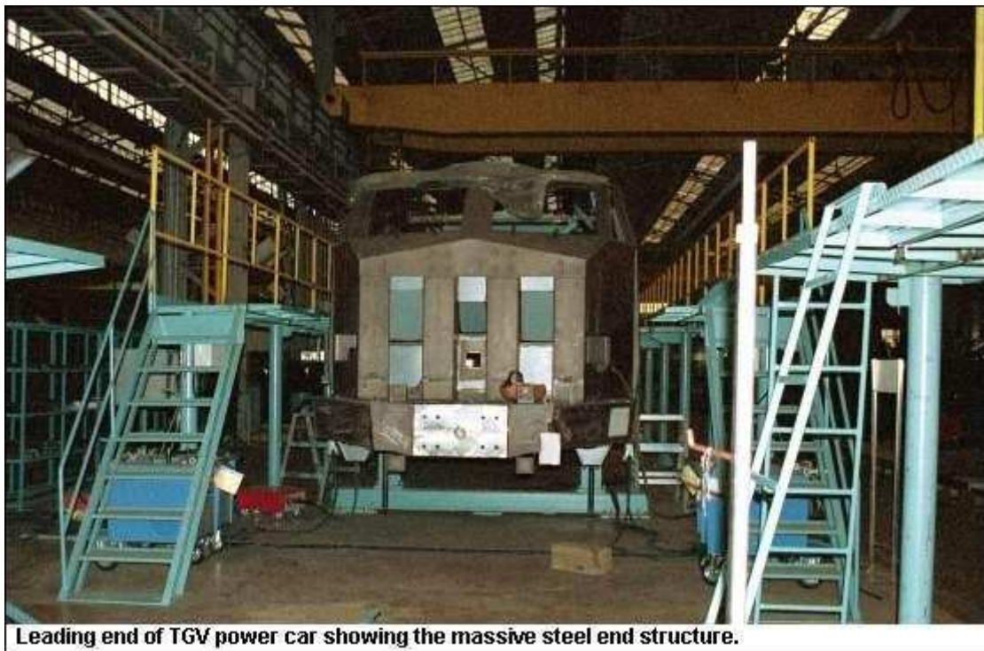
Leading end of TGV power car showing the massive steel end structure.
