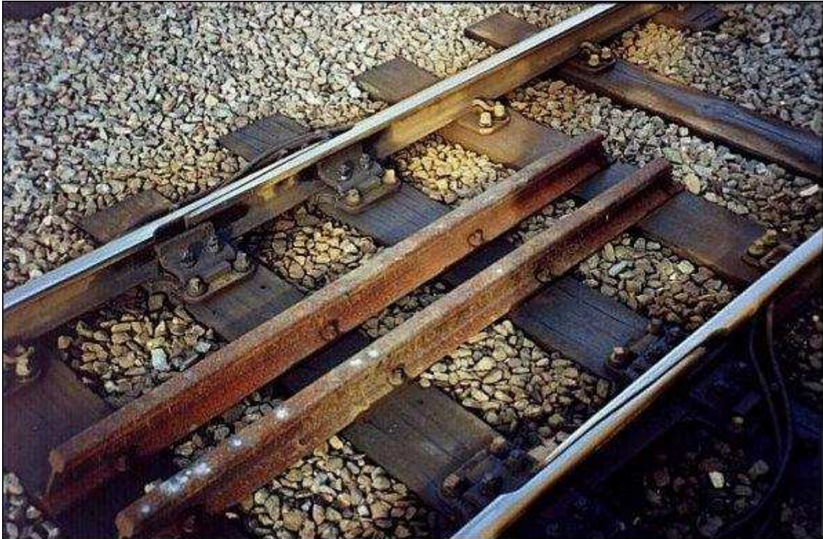
Expansion joints are provided in running rails to allow for temperature changes. The additional rails in the centre of the track are bolted to the sleepers to prevent the sleepers being shifted by rail expansion.
