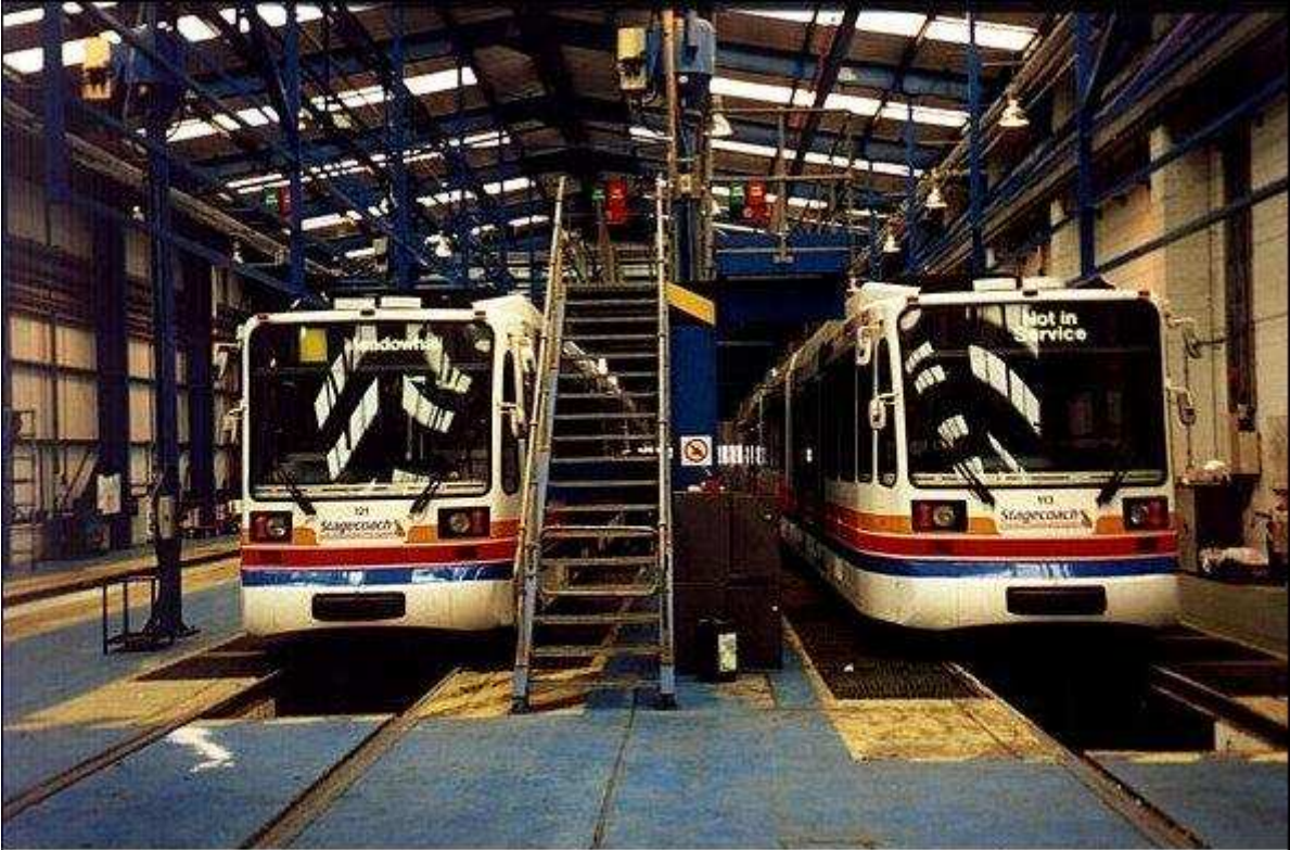
Interior of maintenance depot of the Sheffield (UK) Supertram. Note that overhead walkways are provided to give access to the electrical equipment mounted on the roof. Pits are also provided for under car access.
