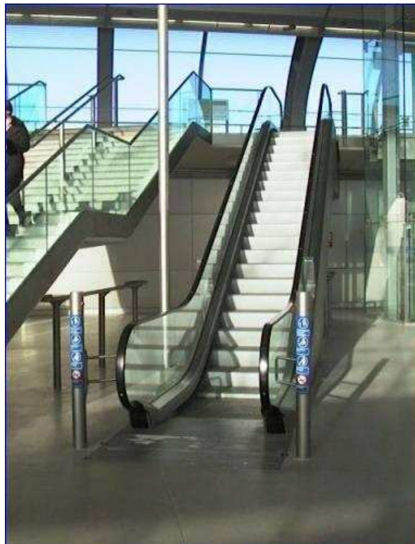
Escalator at Stratford, London, UK. This looks good but it is a very lightweight design, with glass sidewalls and two flat steps at the landings. It is not ideal for heavy use and the glass will need to be cleaned regularly if it is not to look neglected. Note how the ends of the handrails have to be protected by steel pillars.
