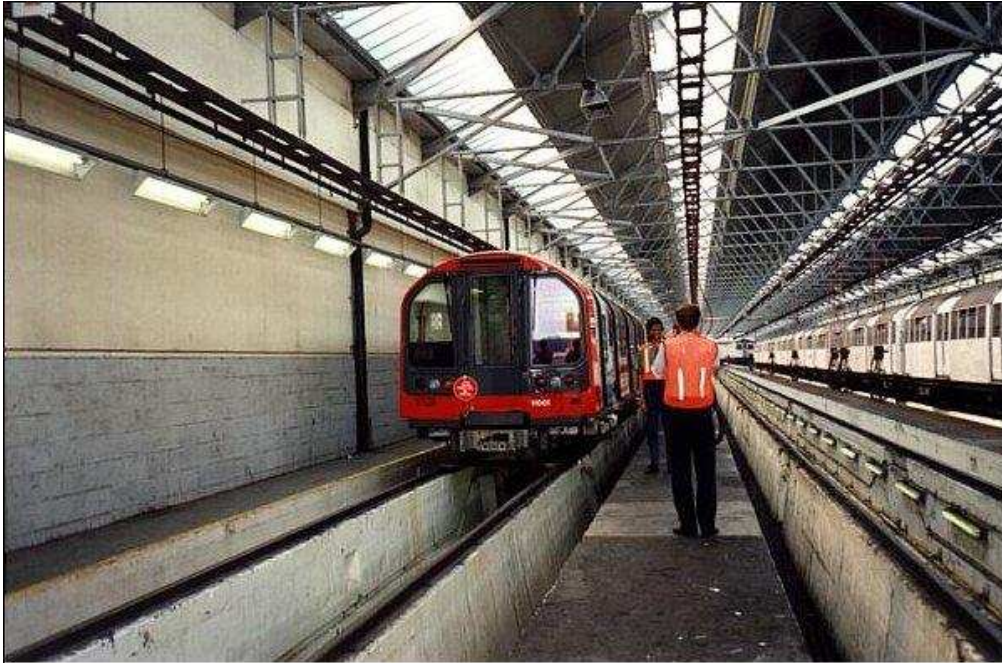
Interior of inspection shed at London Underground's Ruislip Depot showing the centre and side pits provided to allow access under the train. This arrangement would not normally be designed today because of the difficult access and poor natural light..
