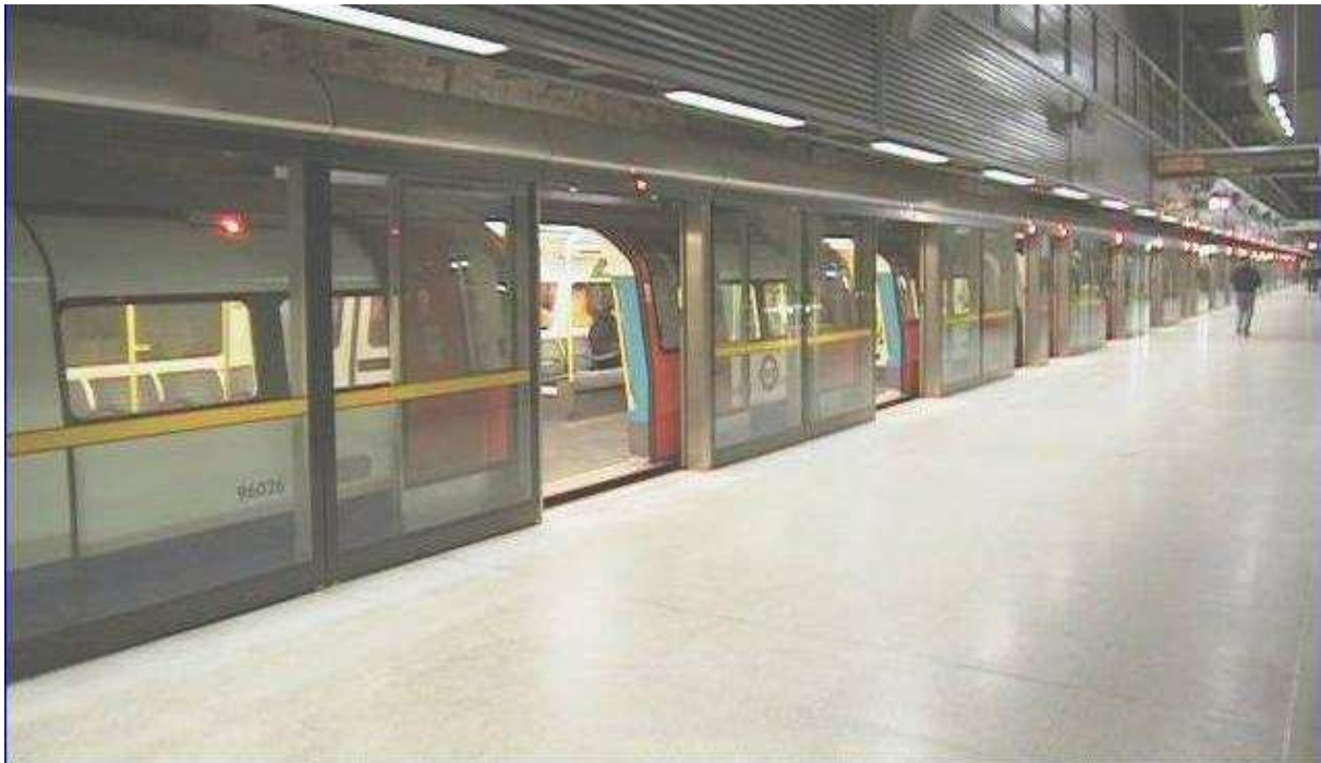
Platform screen doors or Platform edge doors are provided on the new Jubilee Line stations. The operation of the doors is synchronised with those on the train. The driver has to align the train with the doors to within \pm 250 mm in order for the doors to open.
