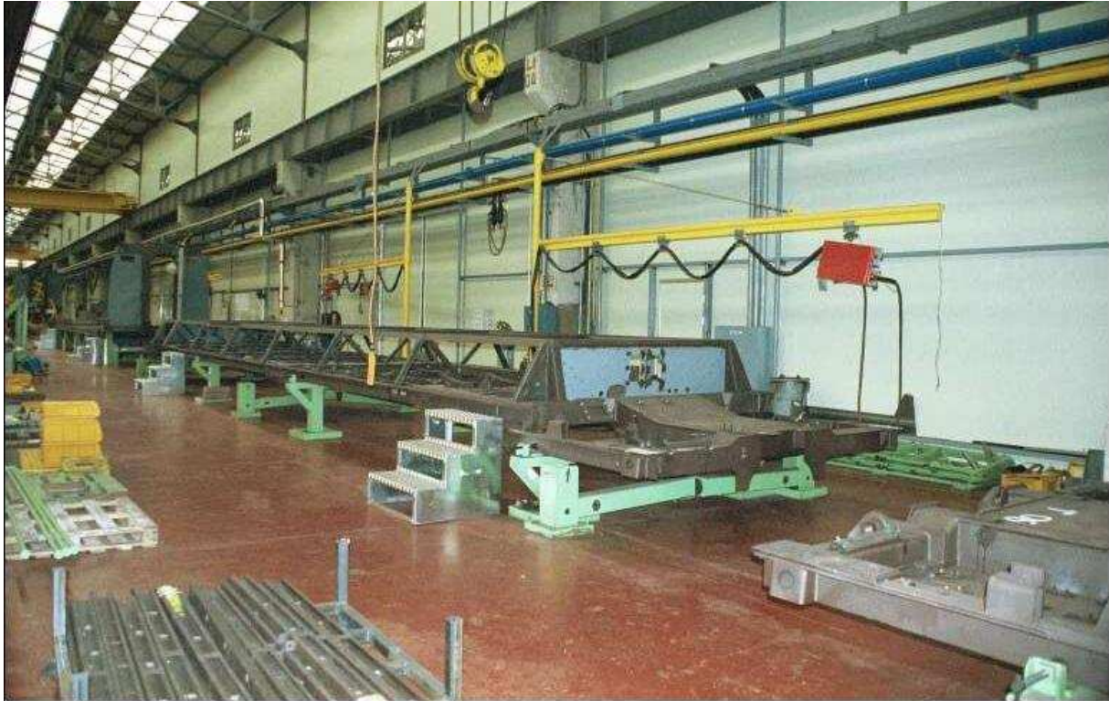
Completed underframe, still inverted where the buffing structure is added
